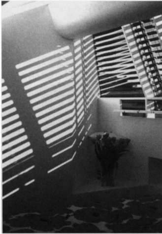
SLATS AT THE WINDOWS OF MURCUTT'S OWN HOUSE CAST SHADOWS THAT CHANGE IN WIDTH AS THE SEASONS TURN. PHOTO COURTESY THE ARCHITECT.
